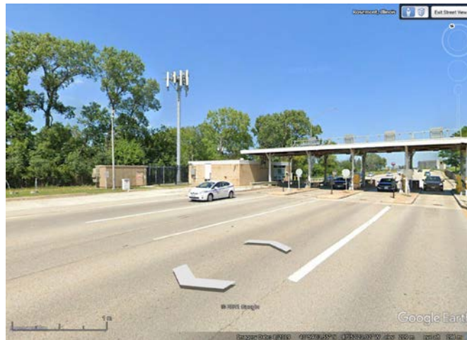
Figure 5-2: Tower Closest to O'Hare Airport (41 59 02 N, 87 52 25 W)
