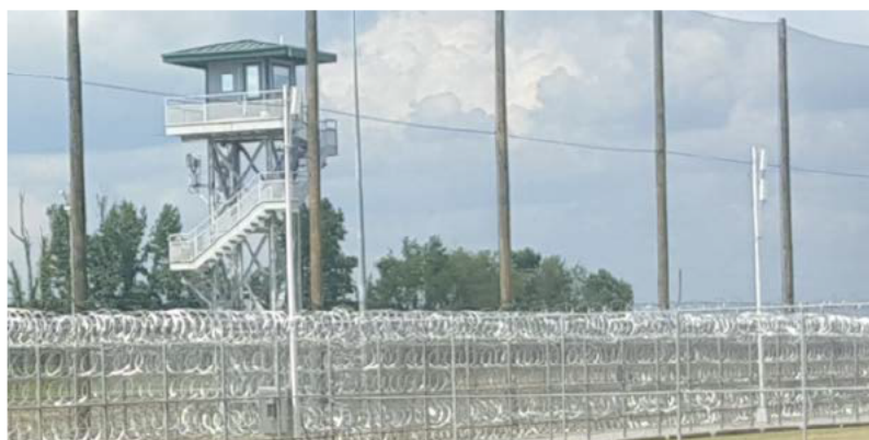
Figure 3-4: Outdoor MAS Installation in “Dog Run”
